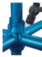
(3) Tightening with a hammer
